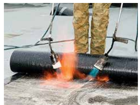
Roof Water Proof
