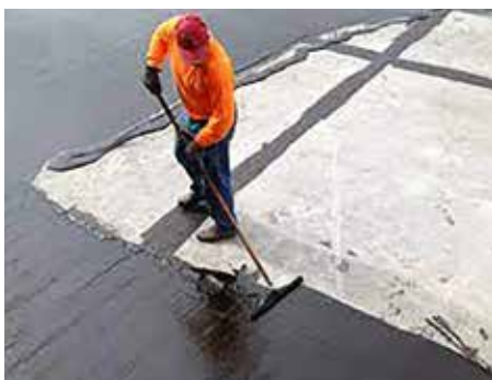
Roof Water Proof
